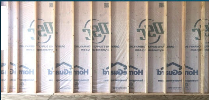
HOUSE WRAP VAPOR BARRIER | P1
