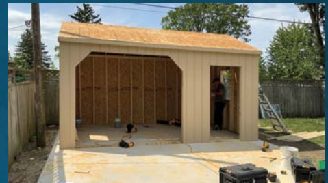
5/8" TONGUE & GROOVE ENGINEERED PANELS
